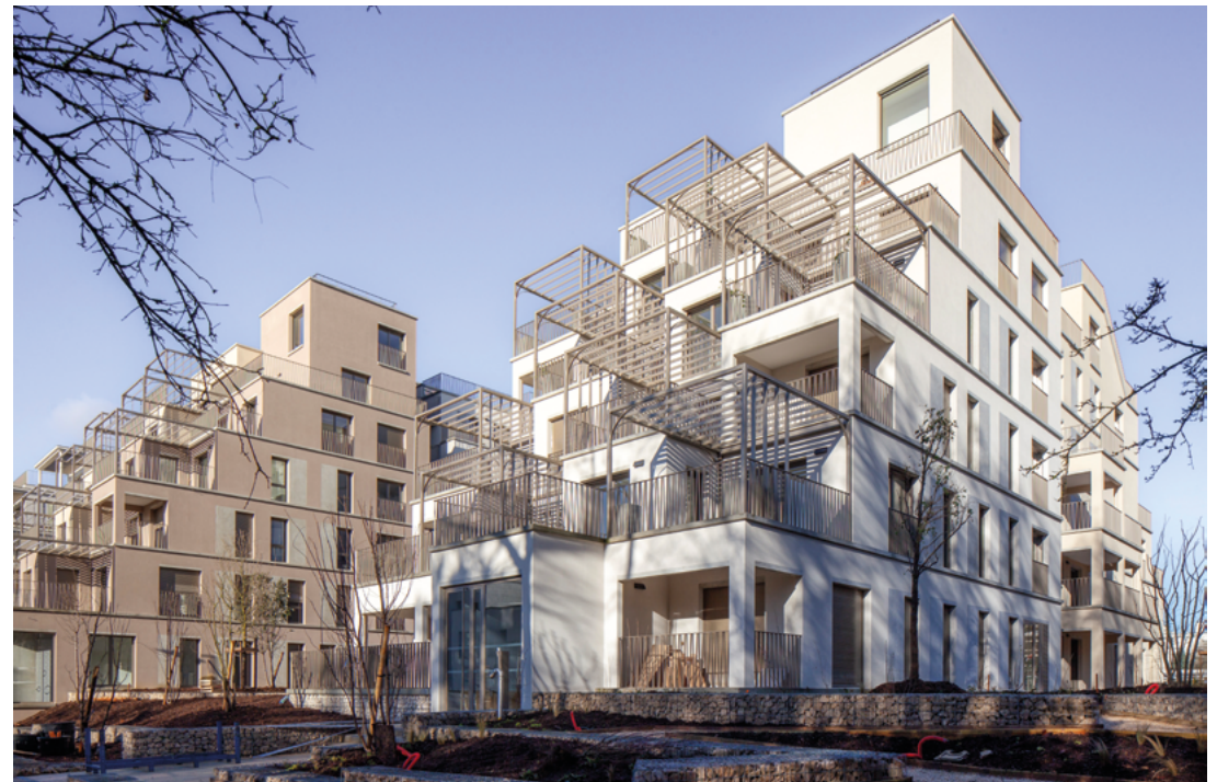
Logements, Rilleux-la-Pape, 2026 © S. Grazia
